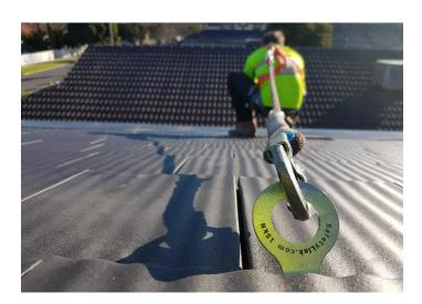
SafetyLink's team designed the TileLink roof anchor (winner of an episode on ABC1 The New Inventors) with unique energy absorbing capabilities, to reduce the risk of injury to the person and damage to the structure.
